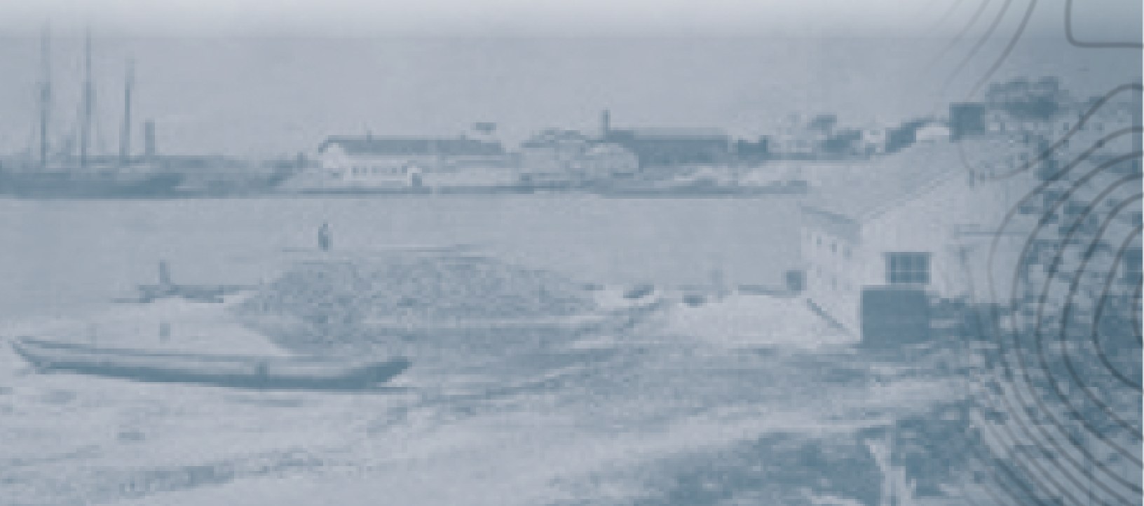
Shell pile in New Haven. Photo: Mystic Seaport Collections.
