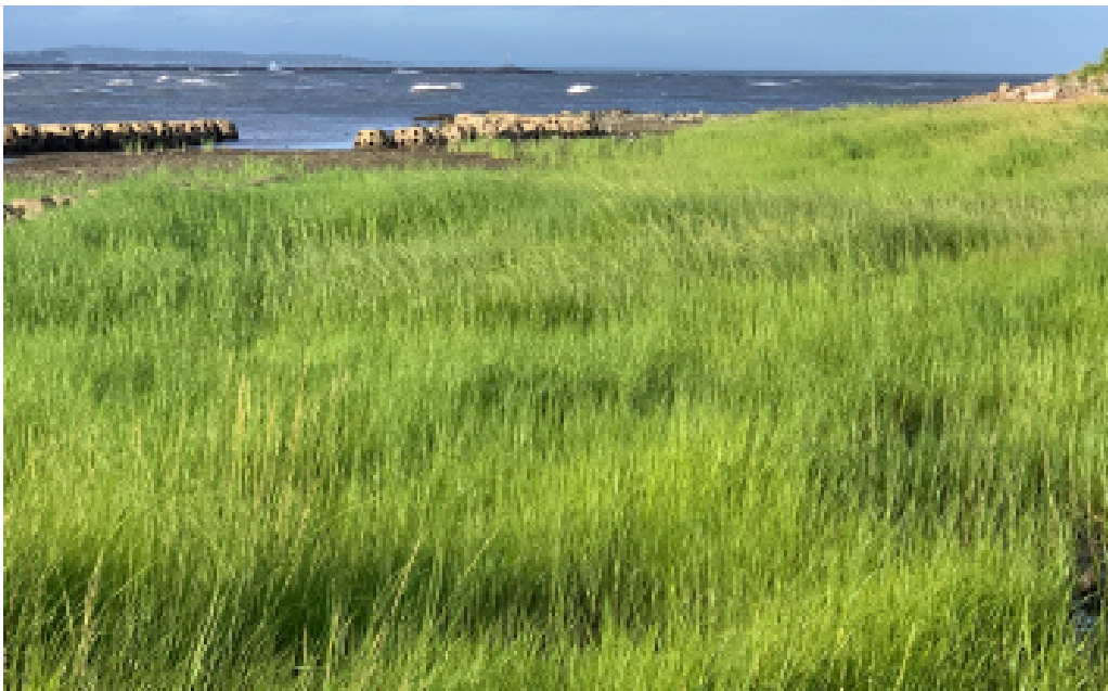
FIGURE 5.13 Stratford Point's Living Shoreline with Reef Balls used as a breakwater protecting the marsh toe and slowly becoming an oyster reef. Photo: Jennifer Mattei
